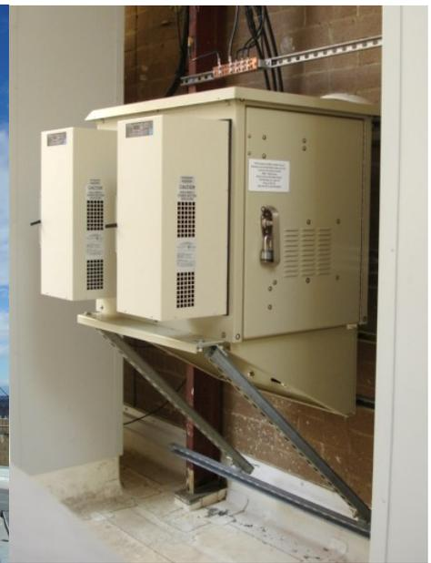
*Equipment cabinet containing transmission equipment for antenna pictured left*
